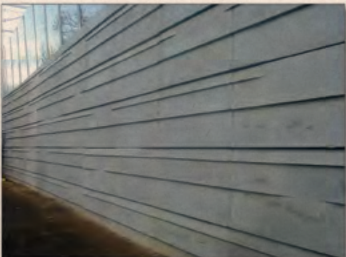
50mm Slopped Pattern at Caulfield - Dandenong Level Crossing Removal + Rail Project Victoria
