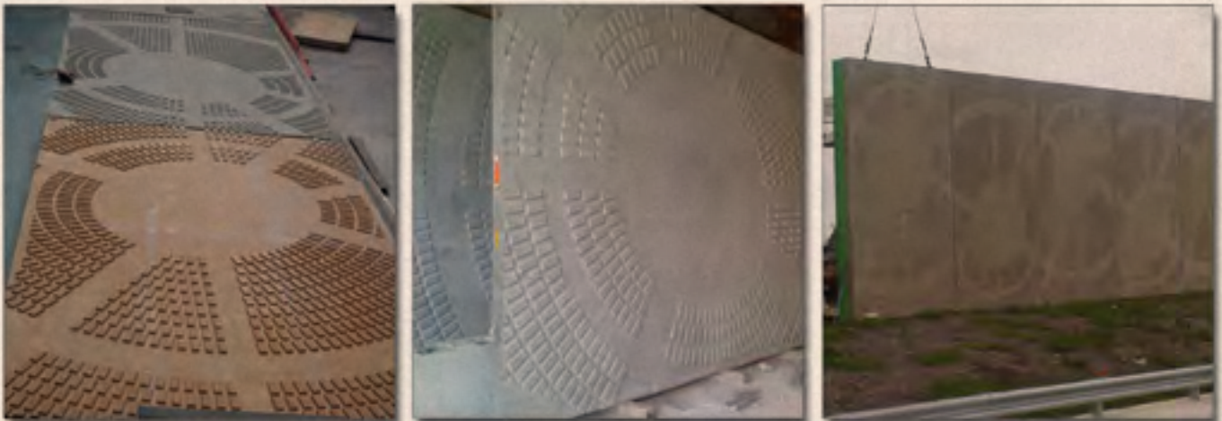
Waverley Park Noise Walls, Monash FWY, Melbourne
