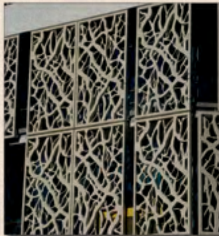
GRC panels at Newcastle courthouse
